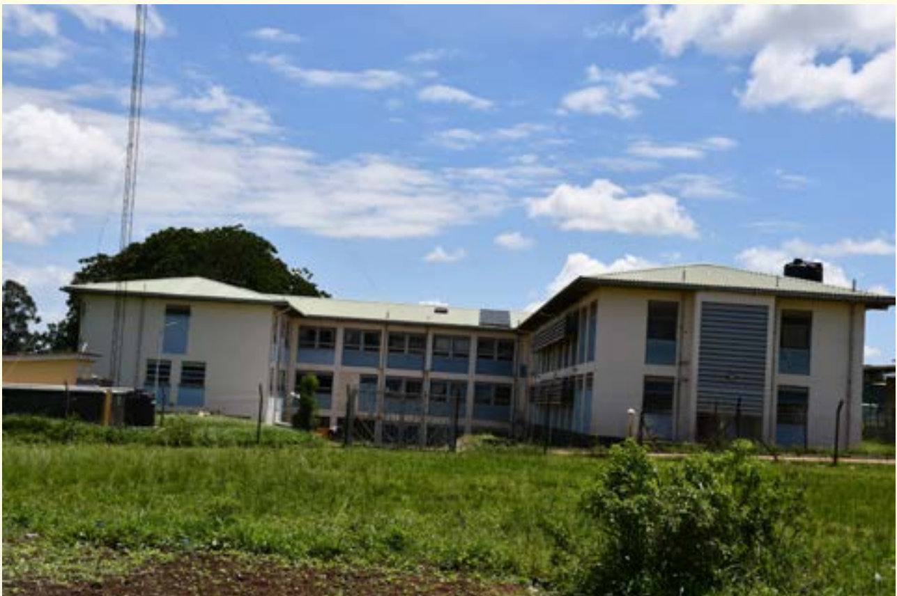
Section of Kiryandongo General Hospital that hosts the mortuary
