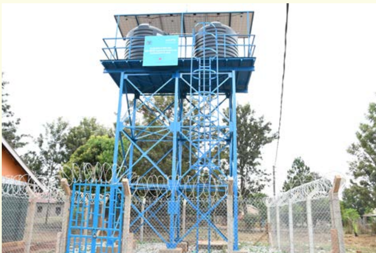
A water reservoir and solar system for supplying piped water at Kigumba COU Primary school
