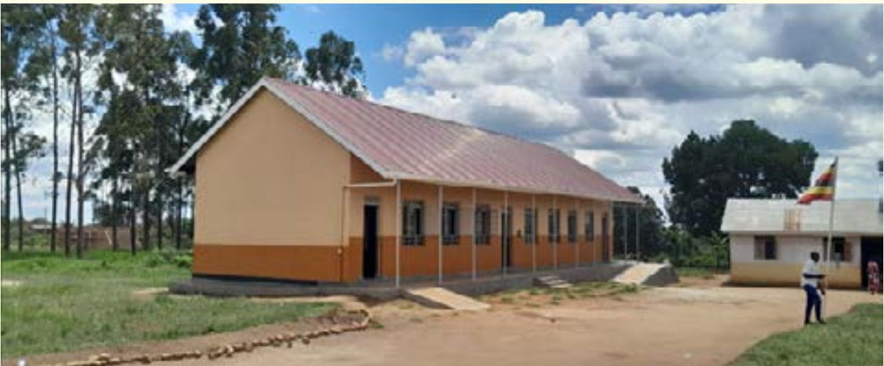
The completed 2-Classroom block at Kyanyi Primary School
